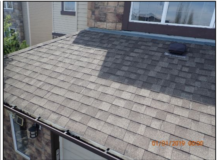
Lower Front and Garage Roof
