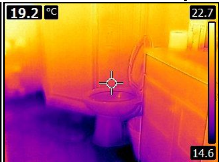
Basement Bathroom - Thermal Image
