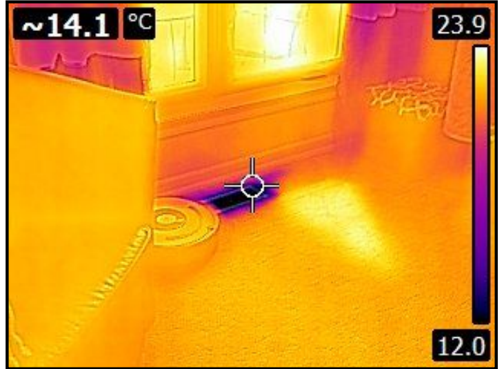
Main Level A/C responding to test at the time of the inspection
