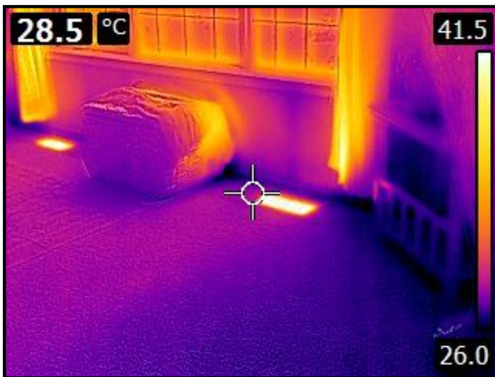
Upper level heating register, responding to test
