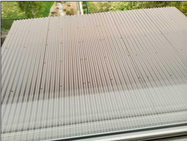
Metal Roof appeared in serviceable condition at the time of the inspection. No prediction of future performance or warranties can be offered.
