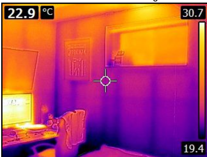
Basement Bedroom - Thermal Image
