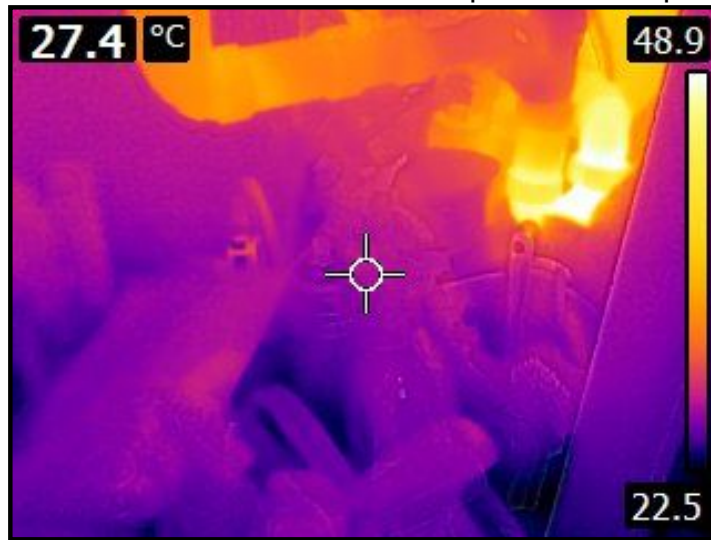
No leaks observed at the time of the inspection.
