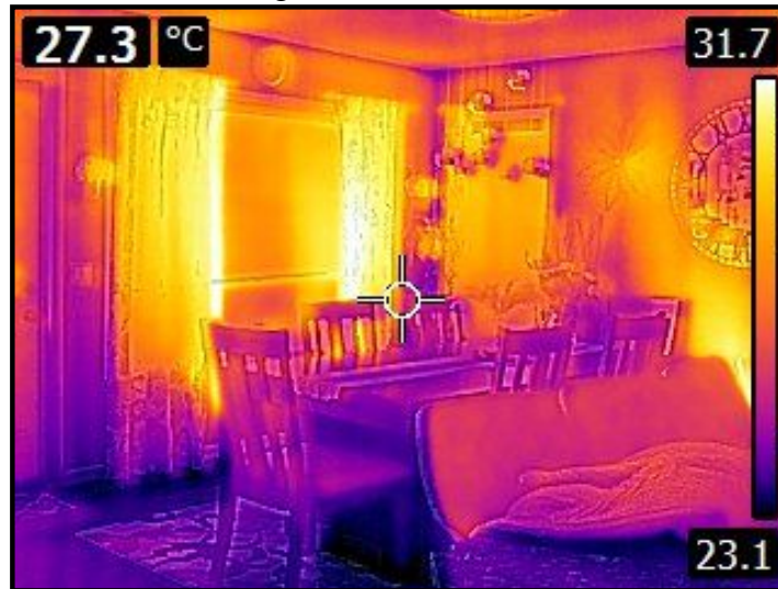
Dining Area - Thermal Image
