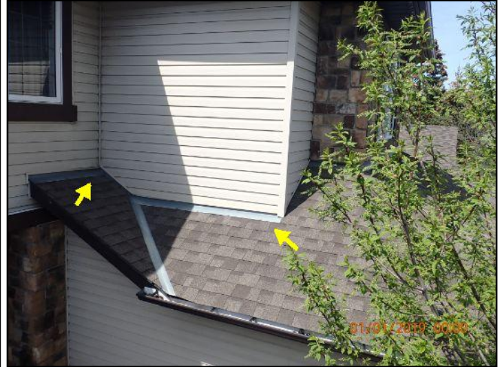
Flashing is fitted and appears in serviceable condition where visible.
