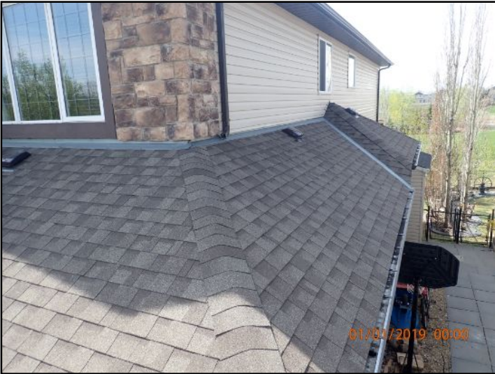
Lower Front Roof
