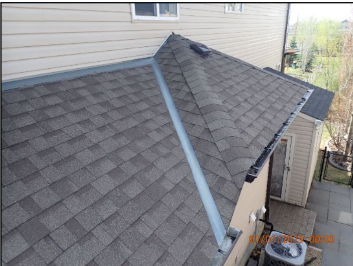
Lower Front Roof
