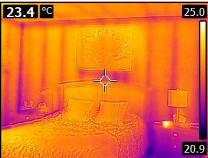
Primary Bedroom - Thermal Image
